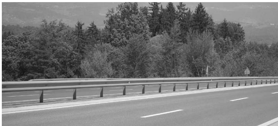
Sl. 1. Jeklena cestna varnostna ograja Fig. 1. Steel road restraint barrier
