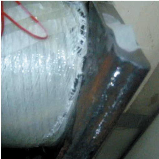
Fig. 14. Failure of the structure in the clamped end under a transverse end load
