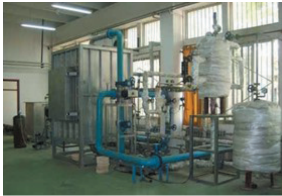
Fig. 3. General view of the research & demonstration TFRR apparatus
